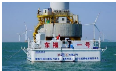
海水无淡化原位直接电解制氢平台 Platform for In-Situ Direct Electrolysis of Seawater without Desalination
