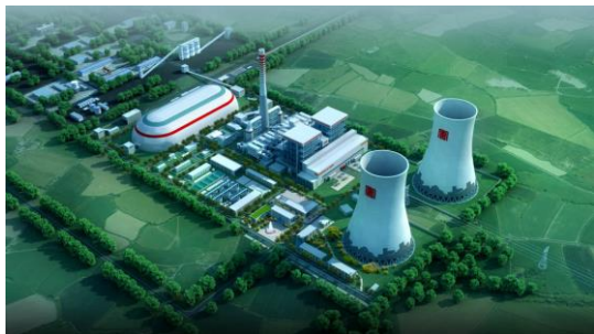
630°C 1000MW超超临界二次再热煤电机组 630°C 1000MW Double Reheat Ultra-Supercritical Coal-fired Power Unit
