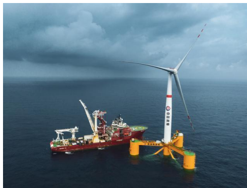
7.25MW漂浮式风电机组 7.25MW floating wind turbine
