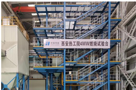
4MW氨/煤混燃试验台 4MW Ammonia / Coal Co-combustion Test Bench
